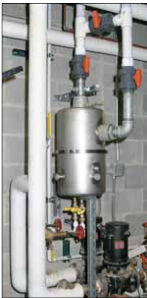
Stainless steel VLS separator installed in a prison facility on a vacuum toilet system.
